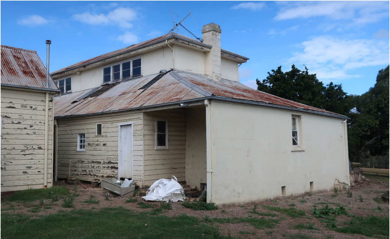
Photo 3-5 The north-west corner of the homestead has a semi-enclosed section leading to a subterranean cool room
