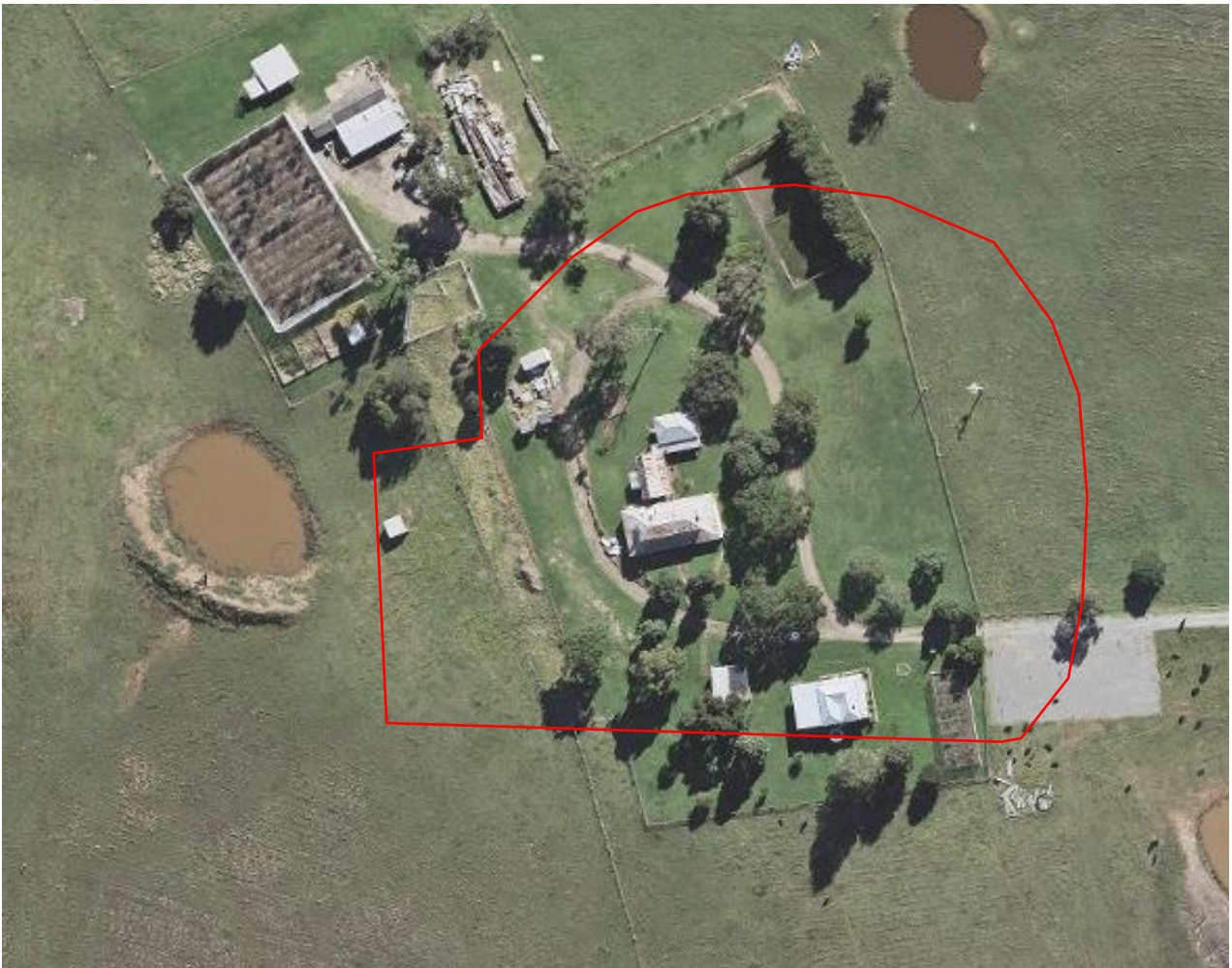
Figure 5-1 The recommended heritage curtilage of Meadowvale
