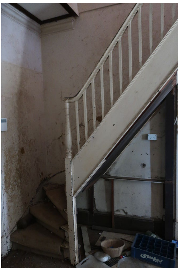
Photo 3-11 The stair is clearly original
