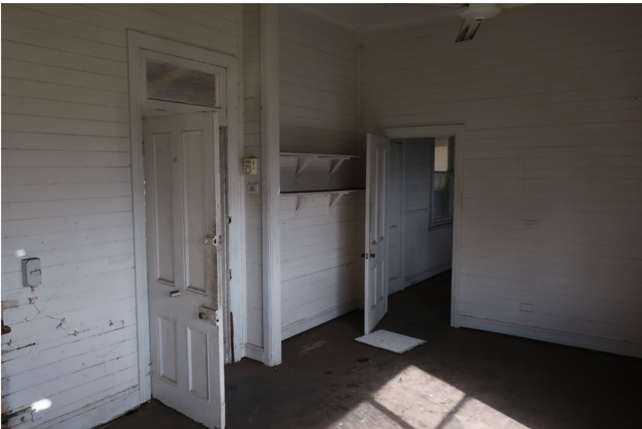
Photo 3-19 Original early Federation doors, pressed metal ceiling and wall cladding in the kitchen
