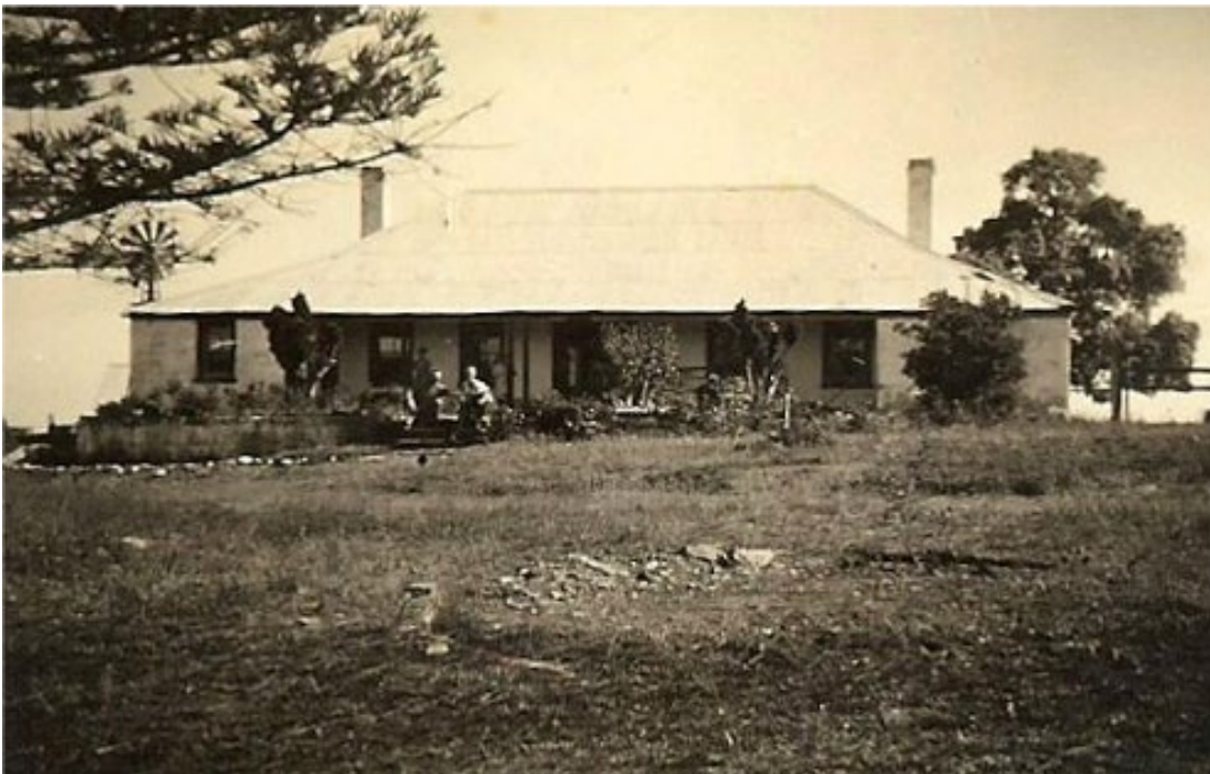
Figure 2-4 Undated c1930 view of the south front of the homestead, showing the front conifers and picket fence gone. The 'Parramatta' arched hoods over the chimneys are gone too
