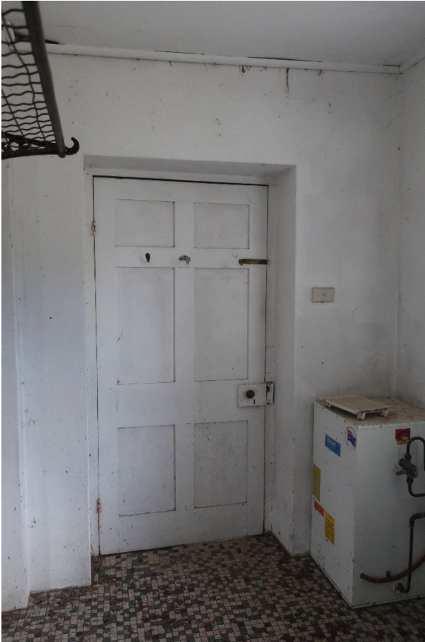
Photo 3-15 A likely original door by the 1960s bathroom fit-out
