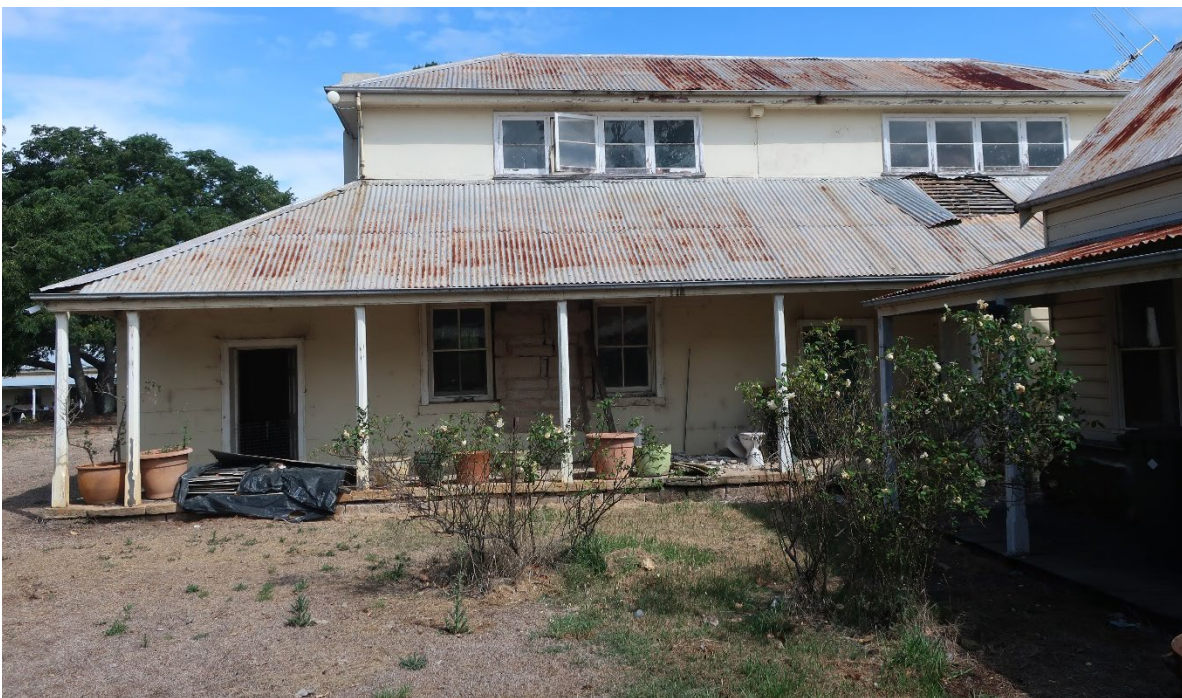
Photo 3-6 The north elevation of the homestead
