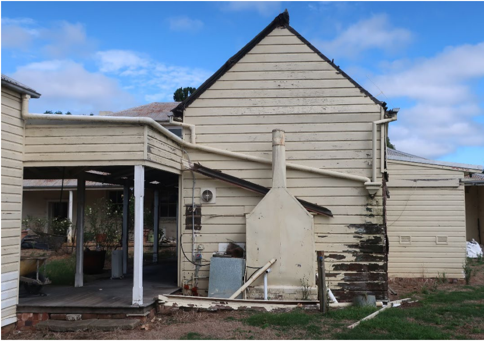
Photo 3-18 The northern elevation of the kitchen building
