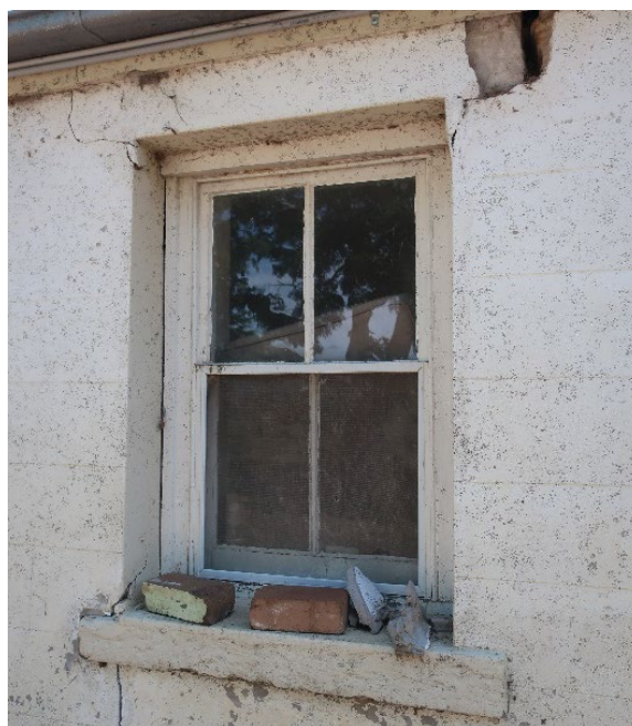
Photo 3-10 A typical original sash window in the east facade
