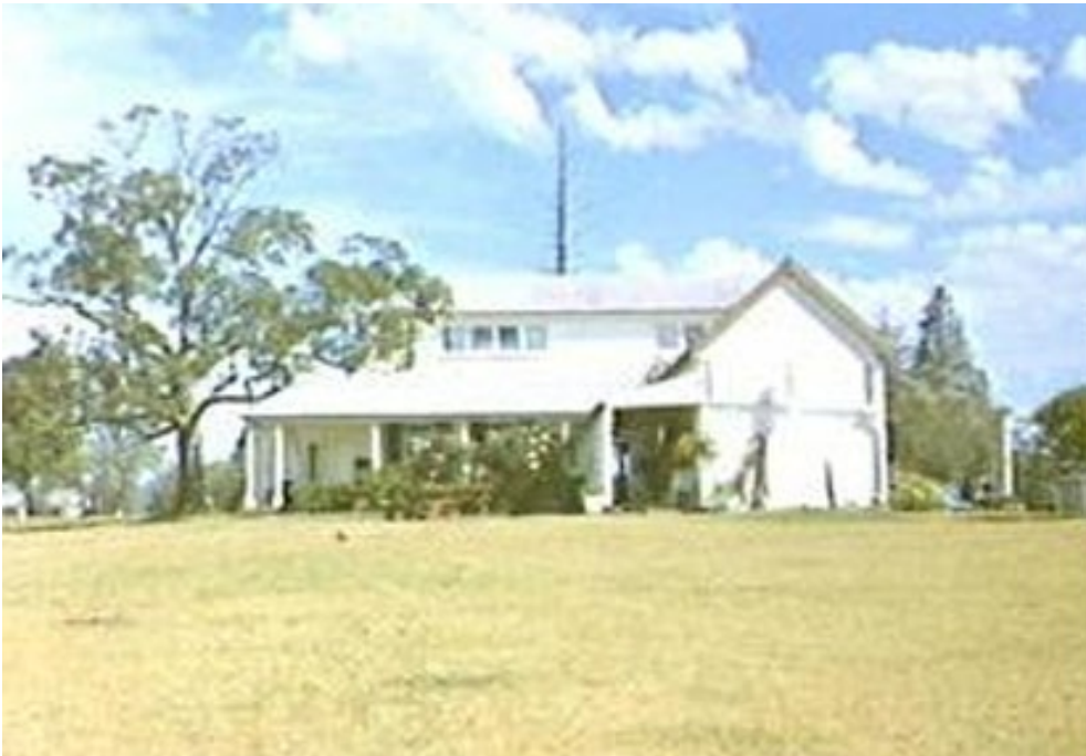
Figure 2-14 1979 view towards the rear of the homestead and northern wall of the kitchen on the right.
