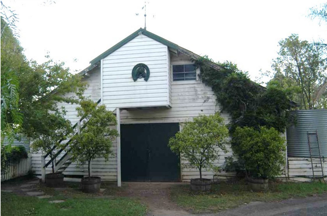
Figure 3-2 The stables, southern front
