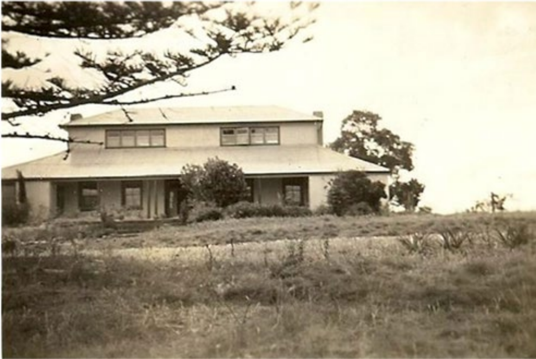
Figure 2-5 Circa 1950 view of the entry front of Meadowvale the homestead. The attic has been extended as a pop-up.
