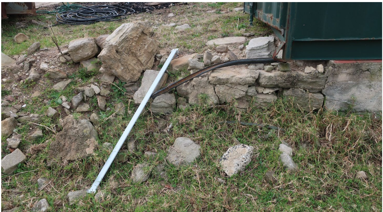
Figure 3-4 Remains of the rough stone cottage following a fire
