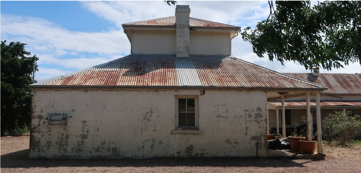
Photo 3-7 The east elevation of the homestead
